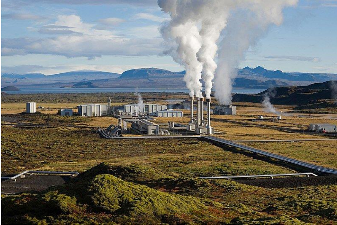
Figure 02: A Thermal Power Station
